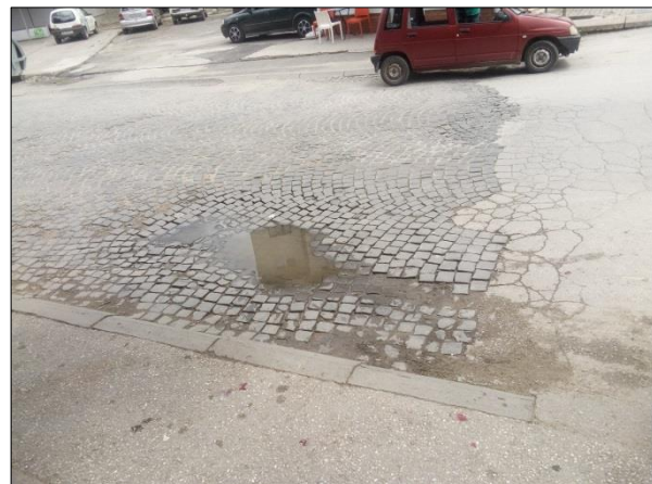
Fig.2 - Current state of the existing street and unformal parking lot across the square (bumpy and destroyed area)
