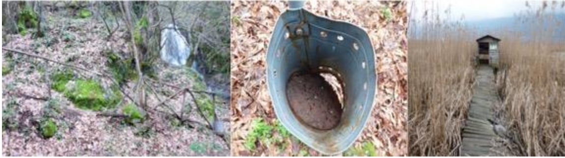
Figure 2: Examples of lack of maintenance of visitor infrastructure around Strumica
